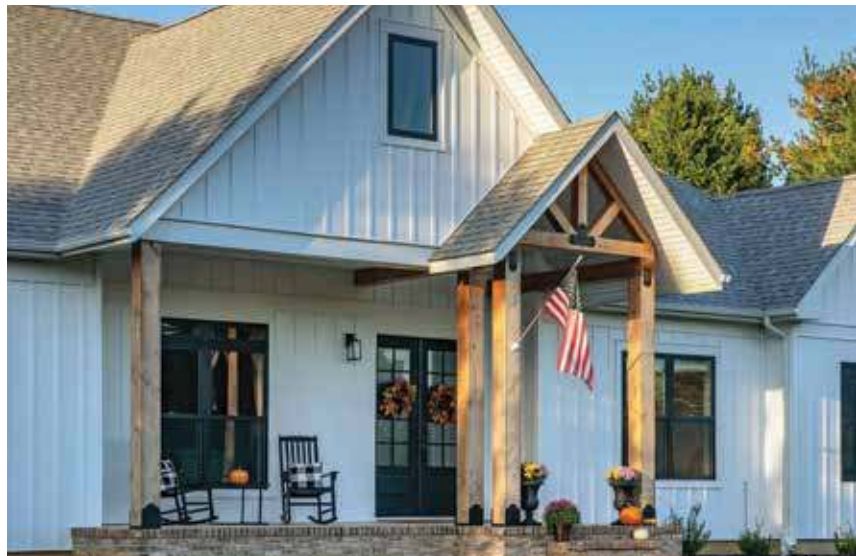
Siding: CedarBoards™ Board & Batten Single 12" in Colonial White.
